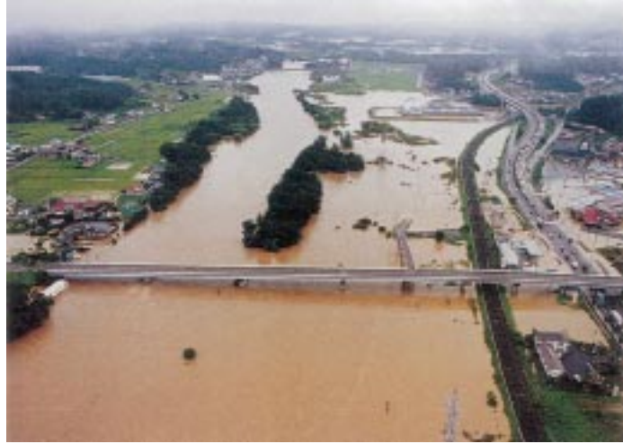
写真4 二本松市両岸の氾濫状況（福島工事事務所提供） Photo 4 Flooded area at the both sides of the Abukuma River in the Nihonmatsu City.
