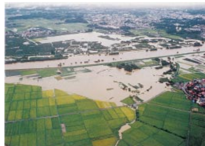
写真9 須賀川市両岸の氾濫状況（福島工事事務所提供） Photo 9 Flooded area at the both sides of the Abukuma River in the Sukagawa City.
