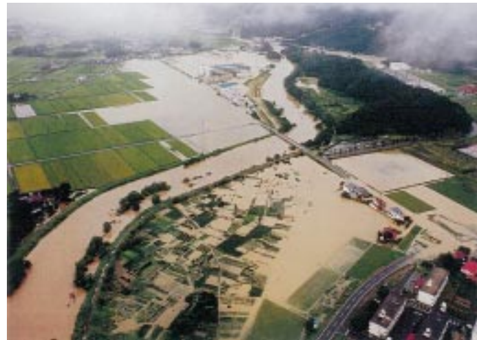
写真5 五百川合流点左岸側の氾濫状況(福島工事事務所提供) Photo 5 Flooded area at the left side of the confluence of the Abukuma River with the Gohyaku-River.
