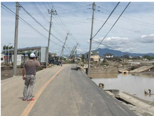
図1 常総市堤防決壊箇所(上三坂地区) Fig. 1 Townscape in the vicinity of Joso City's river breakdown occurrence.
