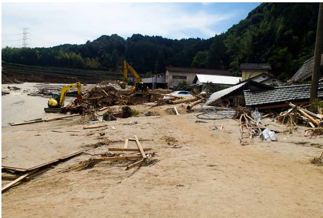
口絵1 多量の土砂と流木の堆積で地形が一変した県道52号杷木松末付近 Fig. 1 Drastic landform change due to accumulate amount of sediment and wood at Hakimasue district, Asakura city, along the prefectural road No.52.
