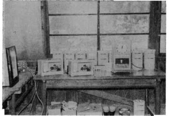
写真-7 隔測受信所全景 Whole view of the signal receiving station.
