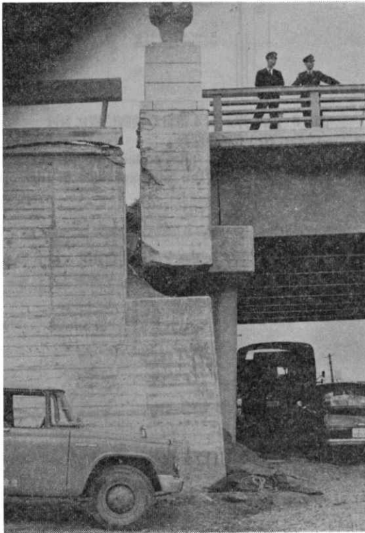
写真—4 昭和大橋左岸橋台の破壊 Damage to the left side abutment of the bridge.
