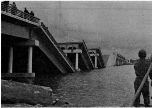
写真-1 落橋した当時の昭和大橋 Five girders of the Showa-Ohashi Bridge fall down into the Shinano River.
