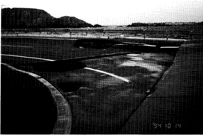
写真16 花咲港東地区の陥没 Photo 16 Depressions (Eastern Area, Hanasaki Port)
