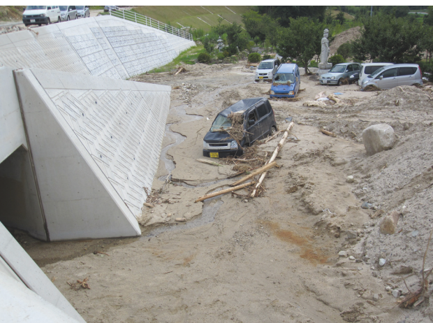
写真6 施設背後の擁壁に設けられた小水路 Photo 6 The water channel was installed at the protection wall of the nursing home Life Care Takasago.
