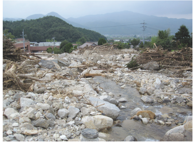
写真7 後背斜面に形成された土石流の流下後の水路 Photo7 Situation of the channel after the flood and sediment disasters on the slope of the facility.
