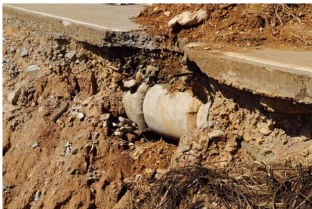
Photo 2 Sewage pipes found buried under the upper portion of the landslide in Kitma.
