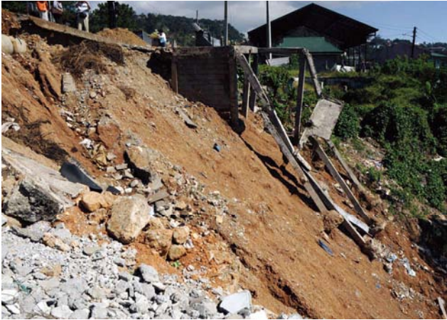
Photo 1 Landslide in Kitma. The house in this photo collapsed down into the slope.
