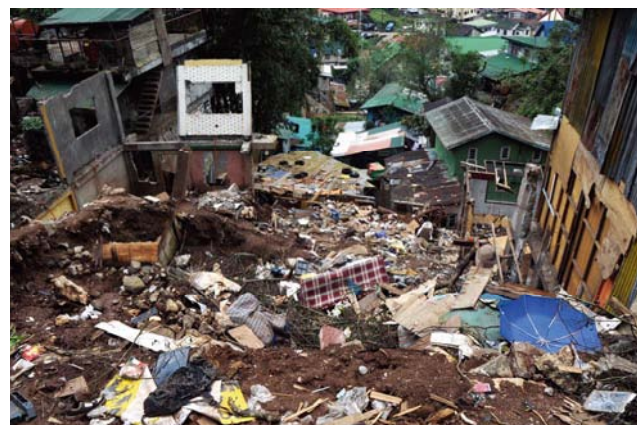
Photo 4 Damage of houses along the slope due to the landslide in Cresencia Village.
