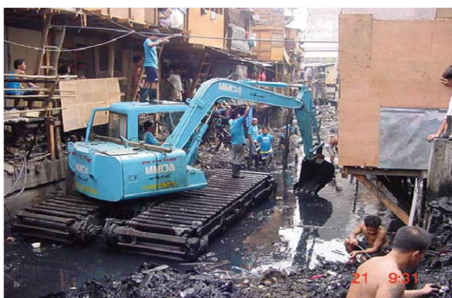
Photo 12 & 13 Dredging urban drainage channels in Metro Manila (Courtesy of the MMDA, 2009).
