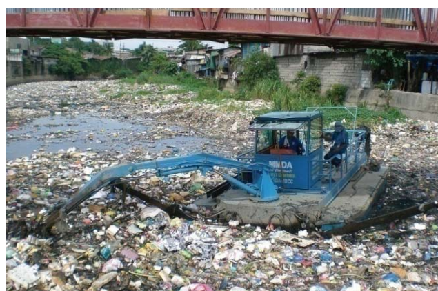
Photo 12 & 13 Dredging urban drainage channels in Metro Manila (Courtesy of the MMDA, 2009).
