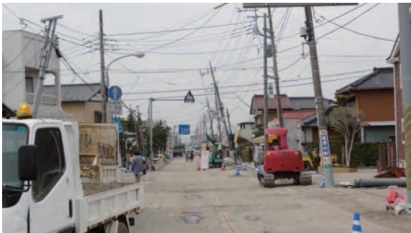
写真10 一帯で大規模な液状化が発生. 多くの電柱が傾いていた(我孫子市布佐). Photo 10 Large-scale liquefaction occurs in the whole area. Many telephone poles are slanted.
