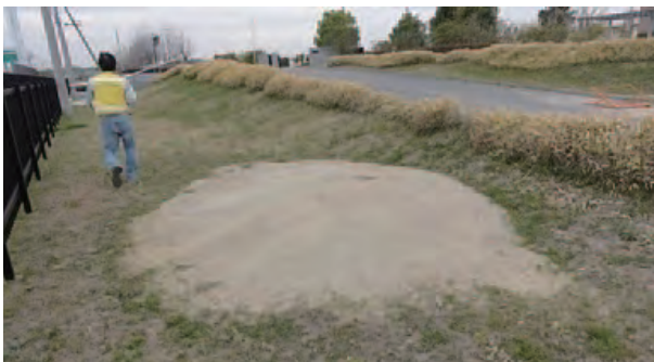
写真11 広範囲に噴砂が発生(下妻市千代川) Photo 11 Sand boil occurs widely (Chiyokawa, Shimotsuma).
