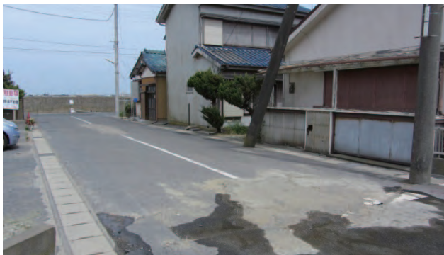
写真5 小規模な噴砂(銚子市大橋) Photo 5 Small quantity of sand boil (Ohashi, Choshi).
