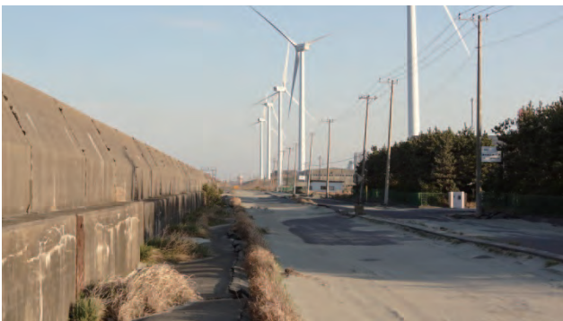
写真4 埋立地における多量の噴砂(鹿嶋市新居浜) Photo 4 A large quantity of sand boil in reclaimed land (Niihama, Kashima).
