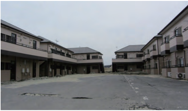
写真2 多量の噴砂と家屋の沈下(神栖市深芝). Photo 2 A large quantity of sand boil and the substance of houses (Fukashiba, Kamisu).
