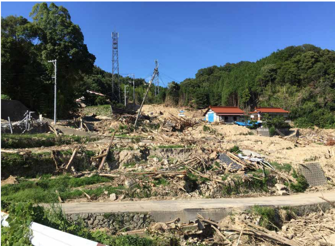
口絵8 安浦町中畑地区の斜面災害。口絵7の矢印地点を地上から撮影。(撮影:2018年8月8日，広島県呉市安浦町中畑) Fig. 8 Landslide in Nakahata District, Yasuura-cho, indicated by the arrow in Fig. 7 photographed from the ground (August 8, 2018: Nakahata, Yasuura-cho, Kure City, Hiroshima Prefecture).
