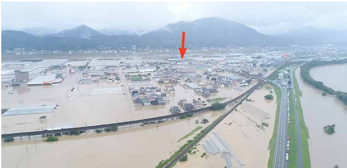
口絵 16 大洲市立図書館(矢印)周辺の浸水状況(撮影:2018年7月7日，愛媛県大洲市東若宮，撮影・提供:大洲市) Fig. 16 Flood damage around the Ozu Library, indicated by the red arrow (July 8, 2018: Higashiwakamiya, Ozu City, Ehime Prefecture; Provided by the Ozu Library).
