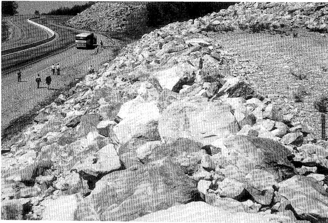
Photo 51 Rock buttresses.
