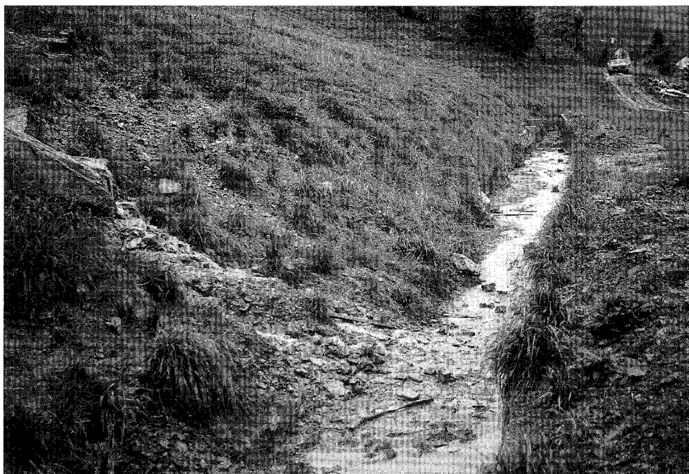
Photo 13 Surface drainage along debris bench.
