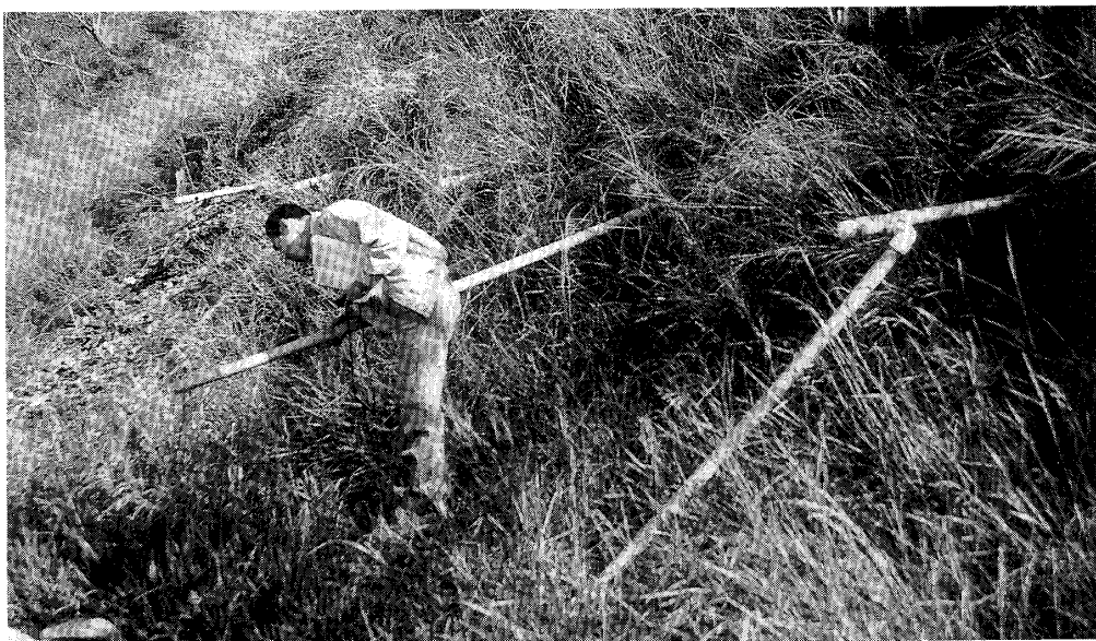
Photo 47 Drainage pipe, Hartford slide.
