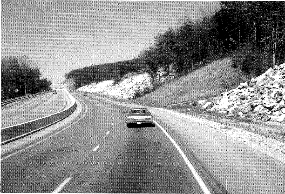
Photo 50 Rock buttresses.
