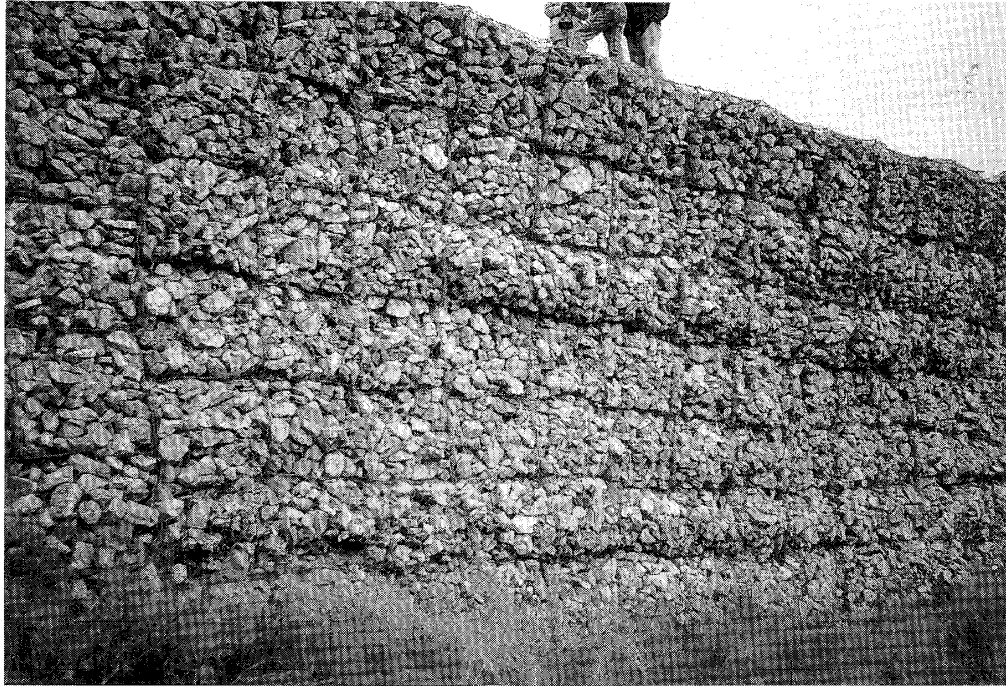
Photo 43 Gabion wall.
