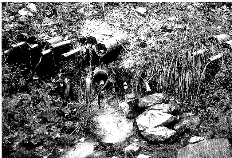
Photo 38 Horizontal drainage.
