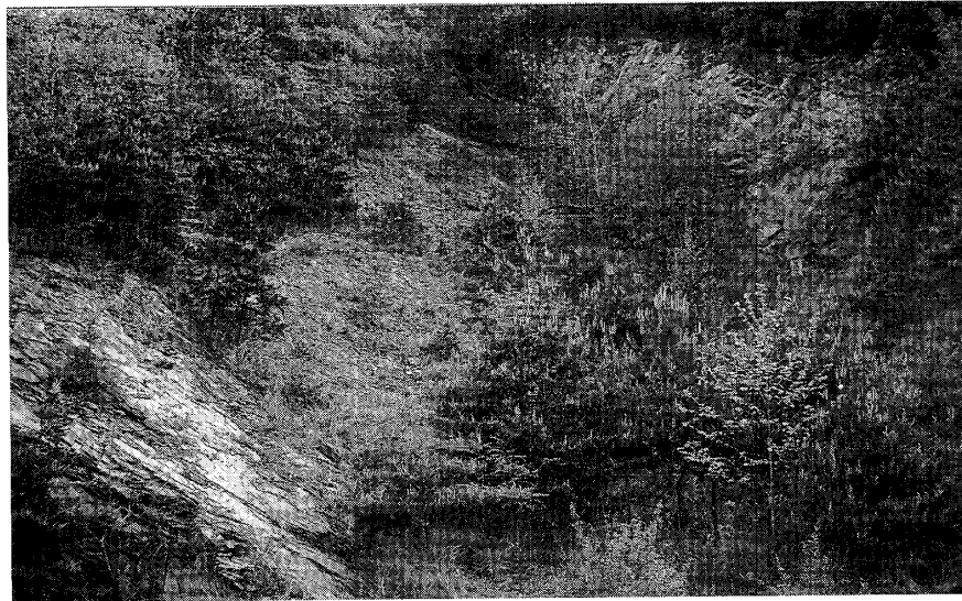
Photo 45 Wedge failure.
