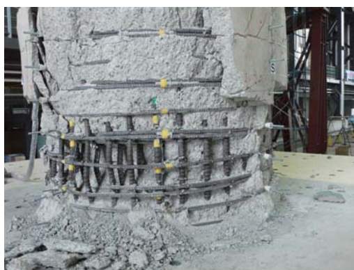
写真 59 C1-5(1)(2)(3)実験終了後南西面 Photo 59 Damage on SW face after C1-5(1)(2)(3) excitations.
