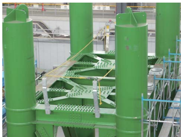
写真 23 端部架台支承設置前 Photo 23 End support before movable bearing was set.
