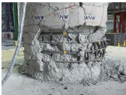
写真 57 C1-5(1)(2)(3)実験終了後北西面 Photo 57 Damage on NW face after C1-5(1)(2)(3) excitations.
