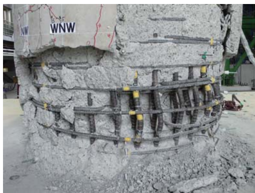
写真 58 C1-5(1)(2)(3)実験終了後西面 Photo 58 Damage on west face after C1-5(1)(2)(3) excitations.
