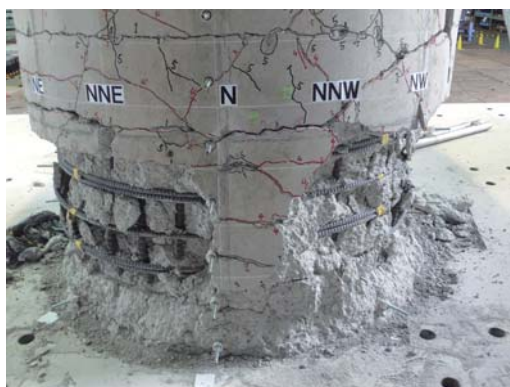
写真 56 C1-5(1)(2)(3)実験終了後北面 Photo 56 Damage on north face after C1-5(1)(2)(3) excitations.
