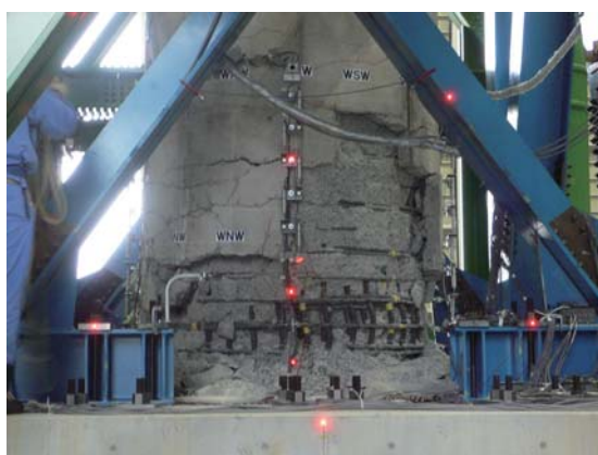
写真 53 C1-5(3)2 回目加振後西面 Photo 53 Damage on west face after C1-5(3)-2 excitation.
