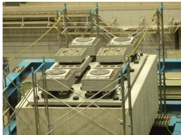
写真 22 RC 橋脚上固定支承仮設置 Photo 22 Set bearings at the column top.
