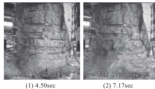
Photo 5.3 Progress of damage at the column base during C1-5(3)-1 excitation.
