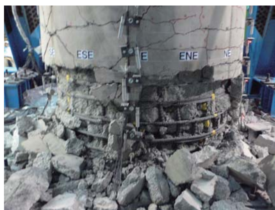
写真 55 C1-5(3)2 回目加振後東面 Photo 55 Damage on east face after C1-5(3)-2 excitation.
