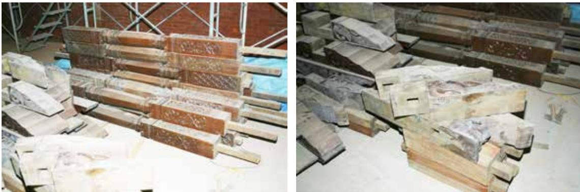
Fig. 2.6 Columns and sub-beams (parts of the replica temple with EXPO 2005 AICHI JAPAN: photo by T. Ohsumi in 2005).
