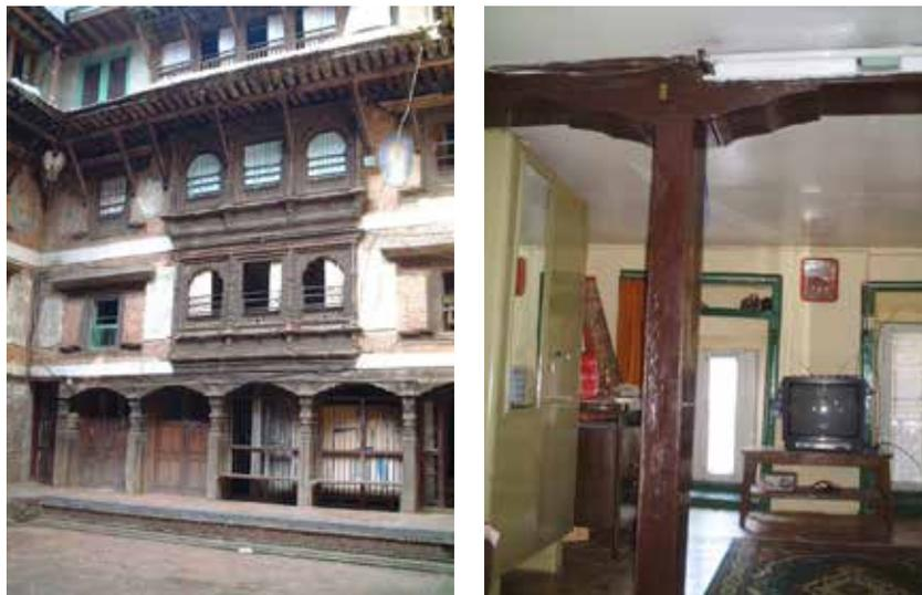
**Fig. 2.9** House's peristyle colonnade and indoor column with a sub-beam in Patan (photo by T. Ohsumi in 2001).
