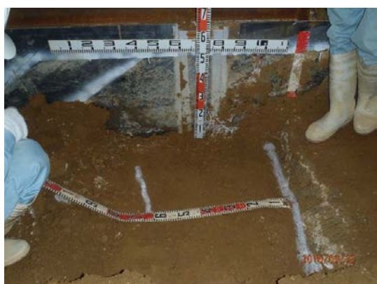
写真 28 シート側天端石灰到達状況 (2) Photo 28 Confirmation of the lime filled into the cracks in the north side of the GCL embankment crest.
