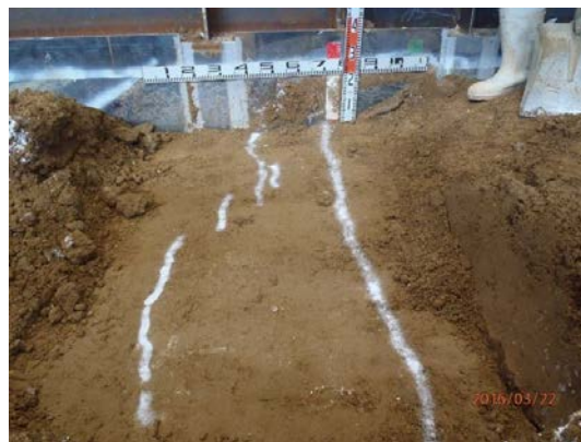
写真 27 シート側天端北側石灰到達状況 (1) Photo 27 Confirmation of the lime filled into the cracks in the north side of GCL embankment crest.
