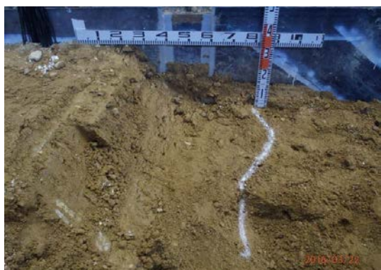
写真 30 シート側天端南側石灰到達状況 Photo 30 Confirmation of the lime filled into the cracks in the south north side of the GCL embankment crest.
