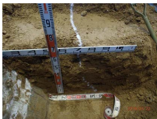
写真 29 シート側天端中央石灰到達状況 Photo 29 Confirmation of the lime filled into the cracks in the center of the GCL embankment crest.
