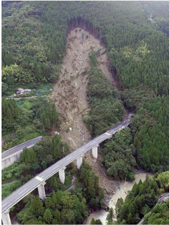
写真1 鳥瞰写真 Photo 1 Bird's eye view of the landslides.
