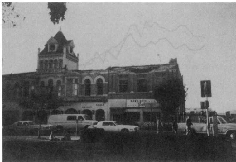
写真6 Watsonville Photo 6 Watsonville
