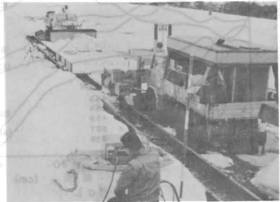
写真1 定置試験装置 Photo 1. General view of stationary snow removal equipment for experiment.
